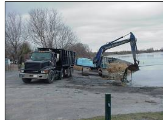
Cleaning up contaminated sediment near Kingston Ministry of the Environment
