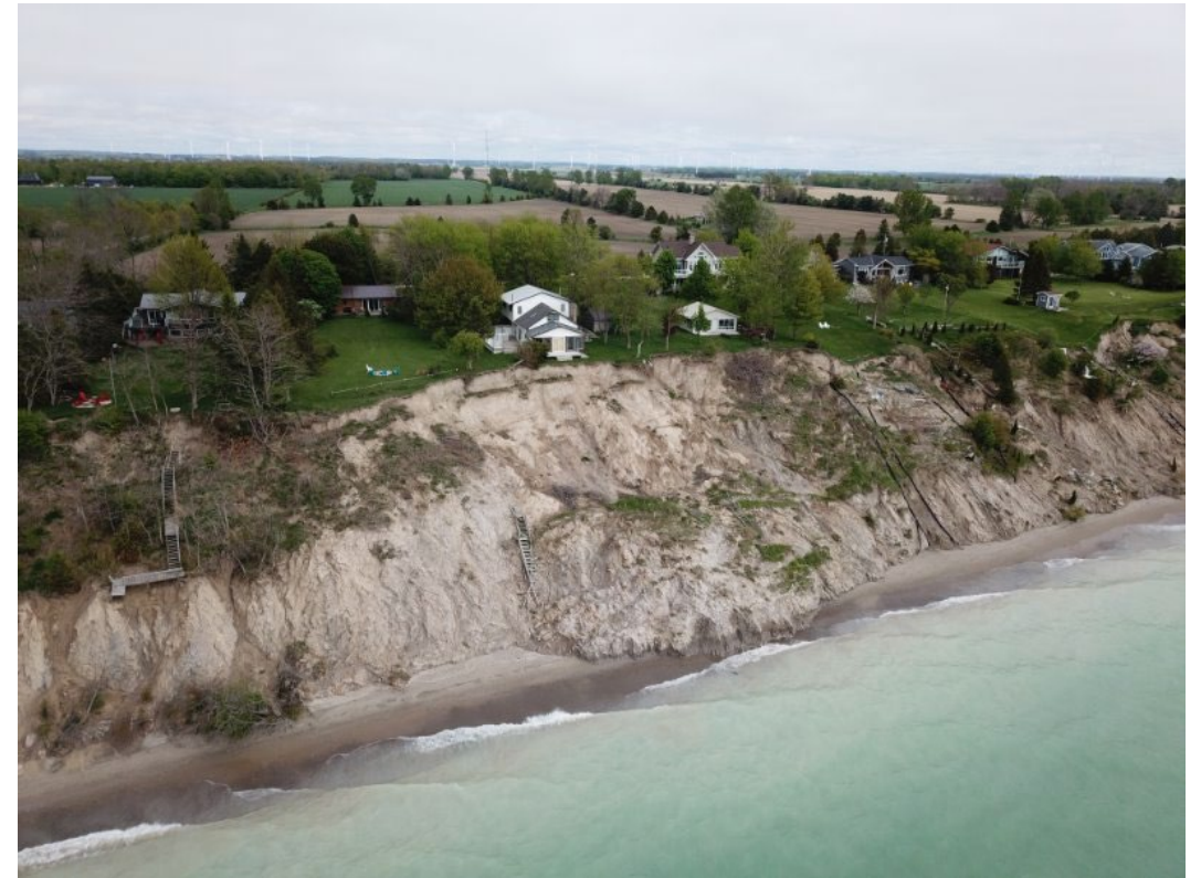
Eroding high-bluff shoreline with evidence of recent slope failure Lake Huron pilot area
